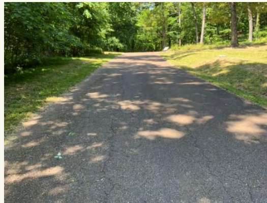
Repair, Rehabilitation, and Reconstruction of Roads and Parking
