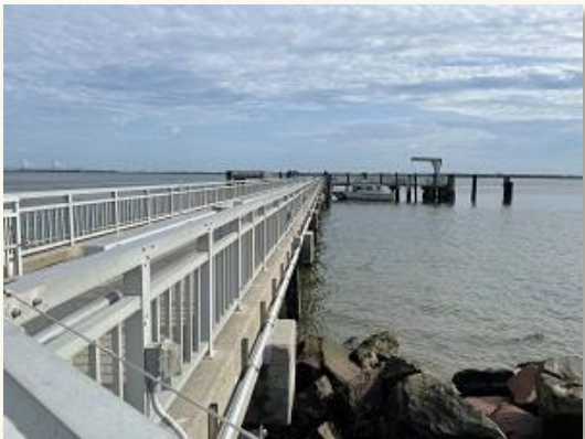
Repair or Replace Docks at Fort Moultrie and Liberty Square
