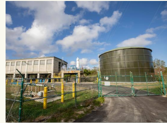
Rehabilitate Parkwide Water and Wastewater Systems
