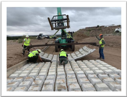
BLM Las Cruces District crews lay out and install articulating mats as part of a GAOA road improvement project. Photo: BLM Las Cruces
