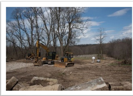
Site of a demolished structure in Cuyahoga Valley National Park, with newly planted trees behind. Photo: NPS/Tim Fenner
